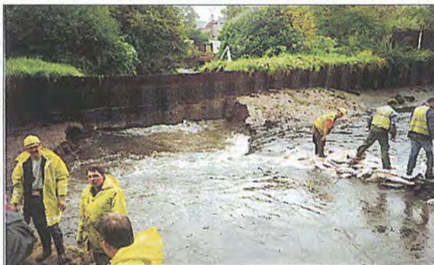
Plugging the culvert.
